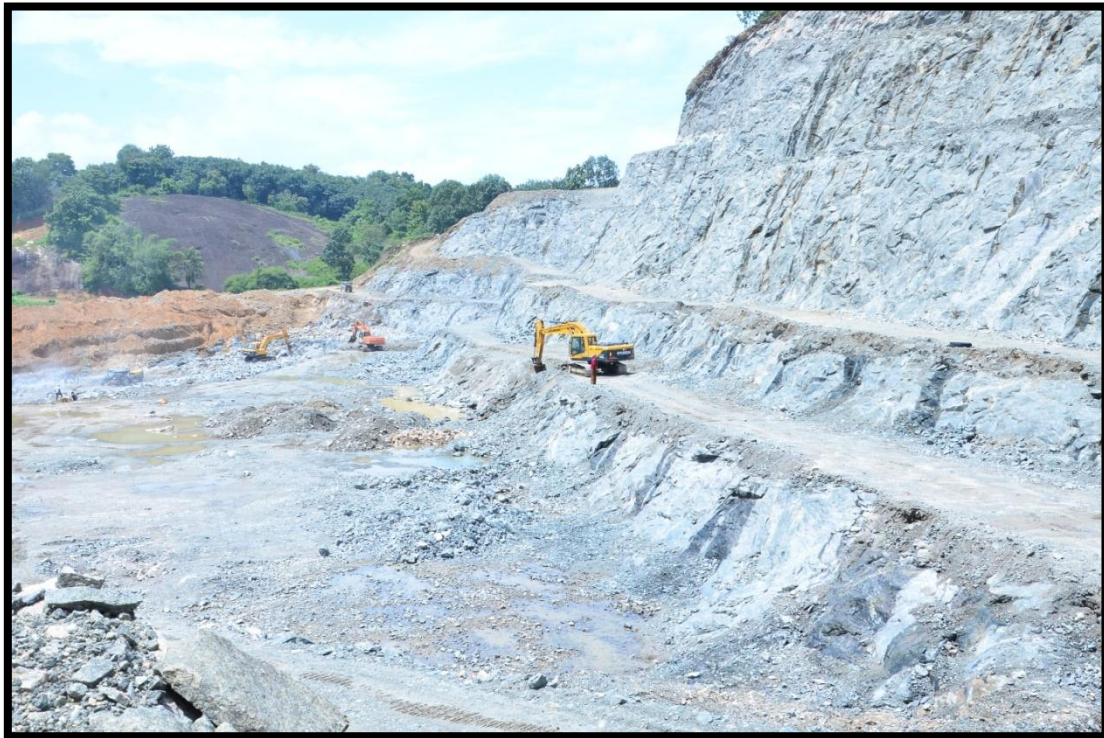
Benches under progress
