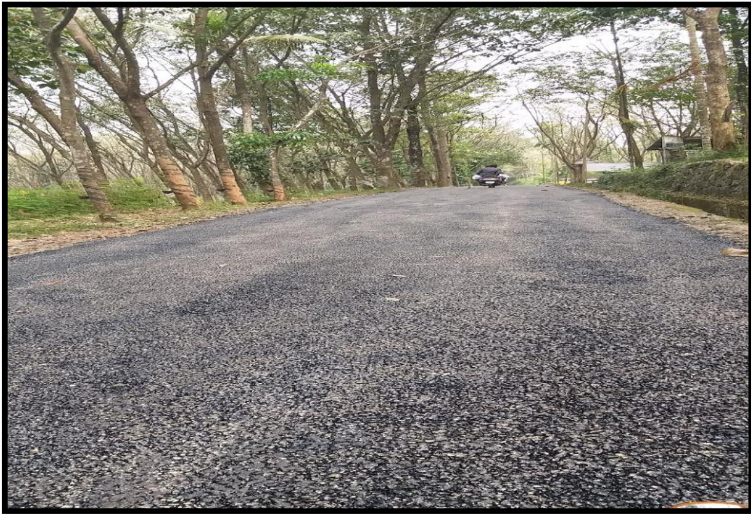
Tarred road to the quarry
