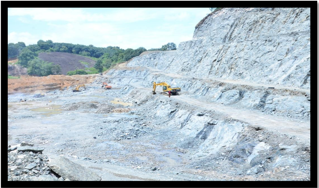
Benches under progress
