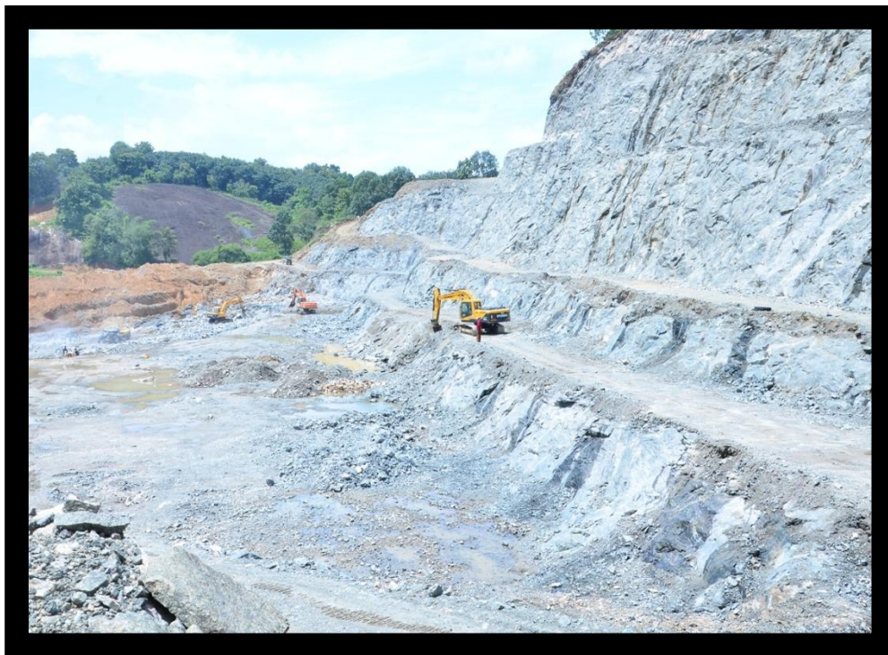
Benches under progress
