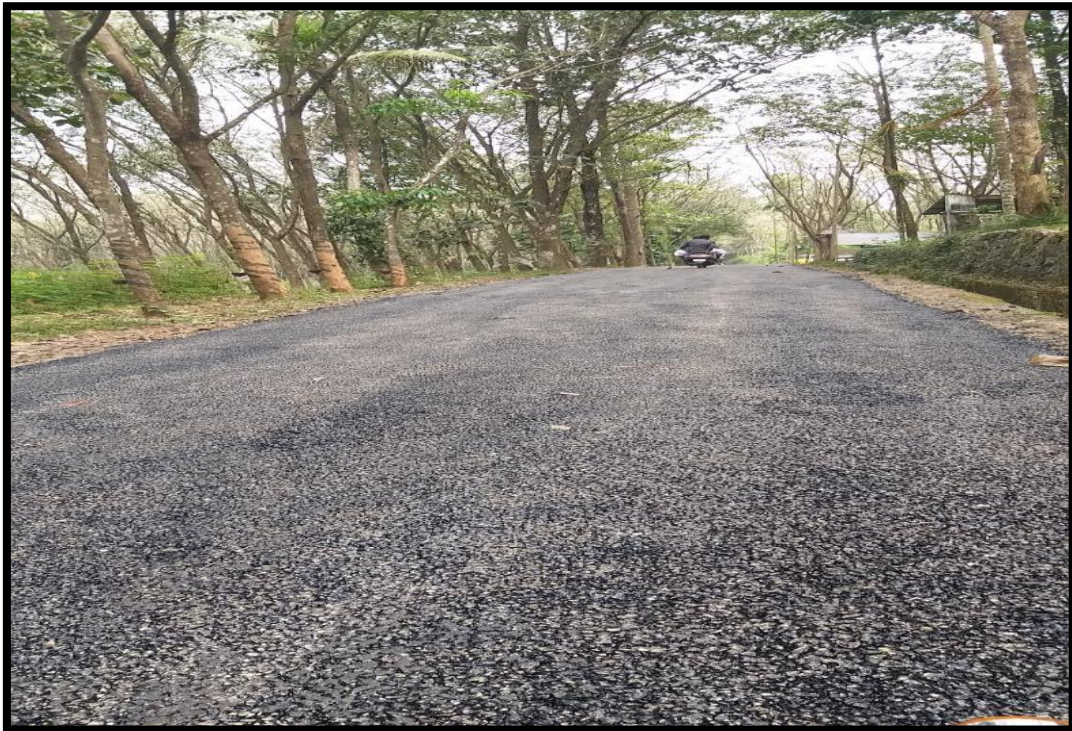
Tarred road to the quarry
