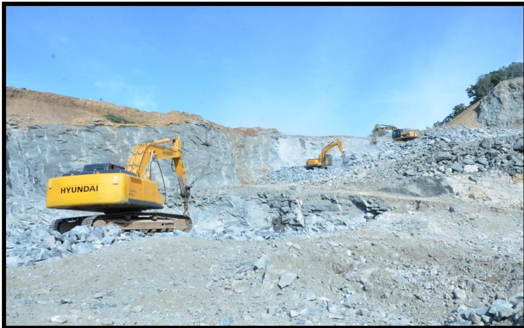
Benches under progress
