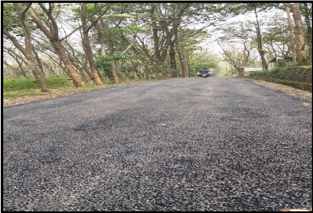
Tarred road to the quarry
