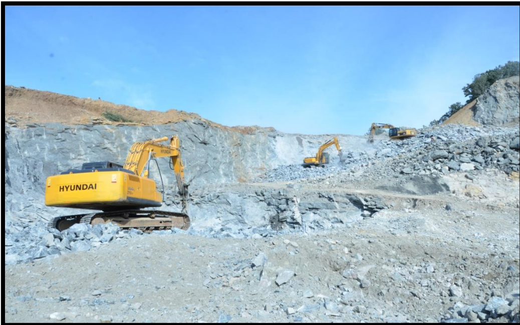
Benches under progress
