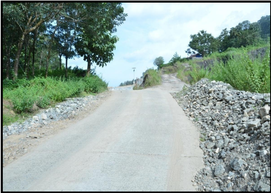
Concreted road to the quarry
