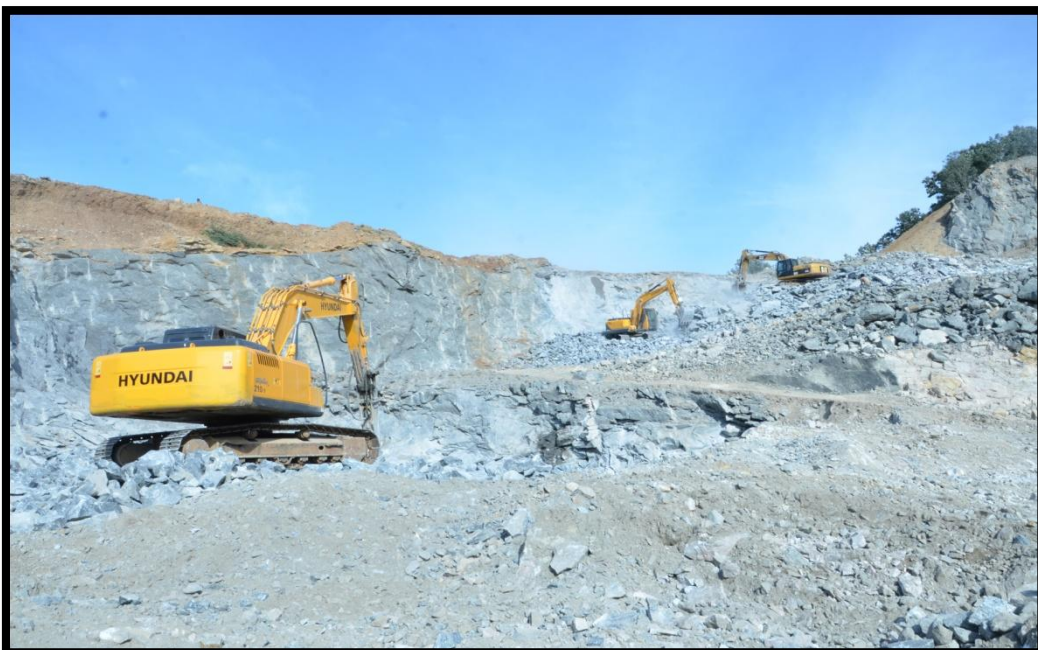
Benches under progress
