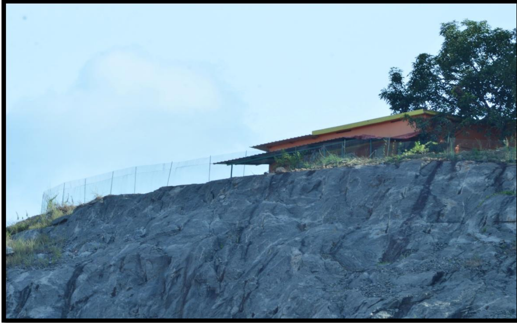
Fencing around the mining area
