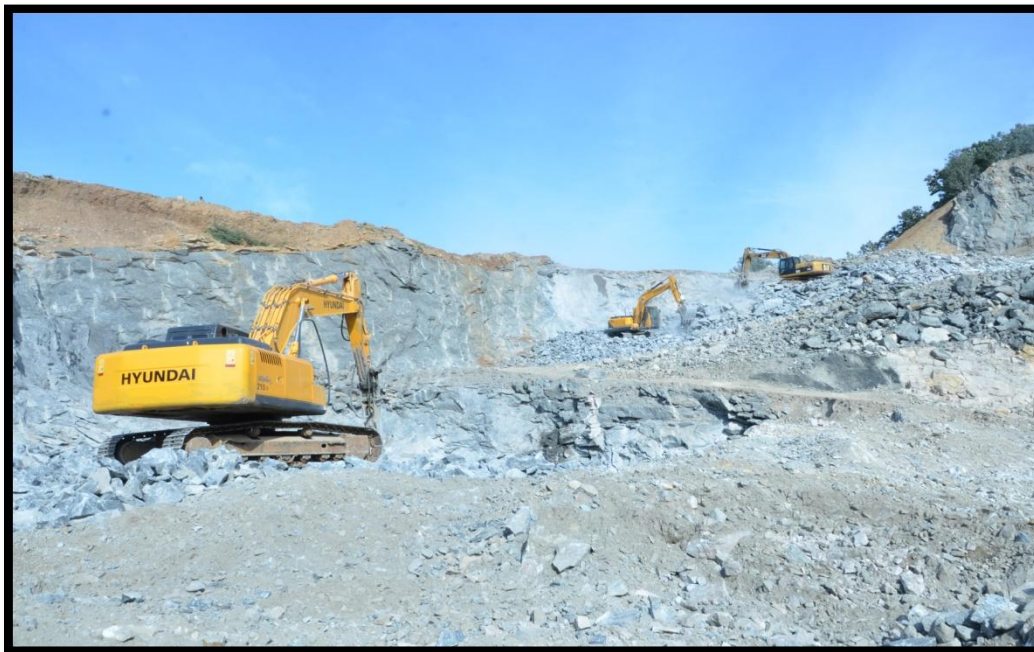
Benches under progress
