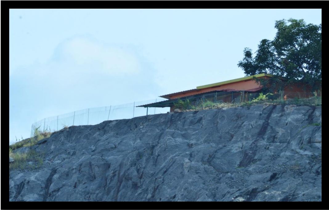
Fencing around the mining area
