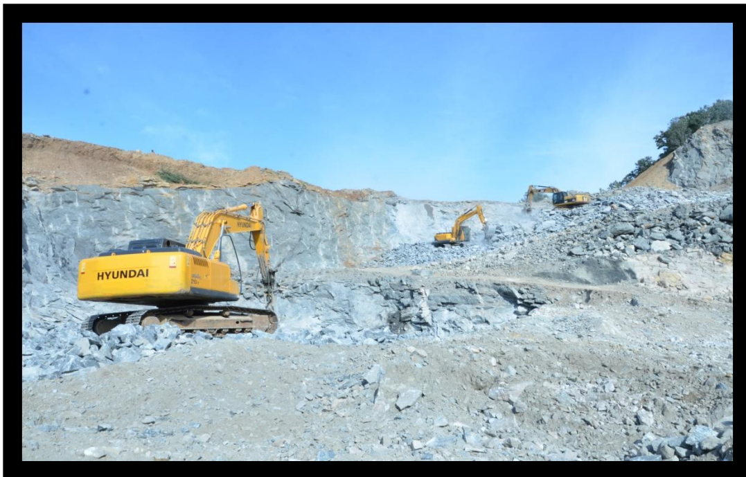
Benches under progress
