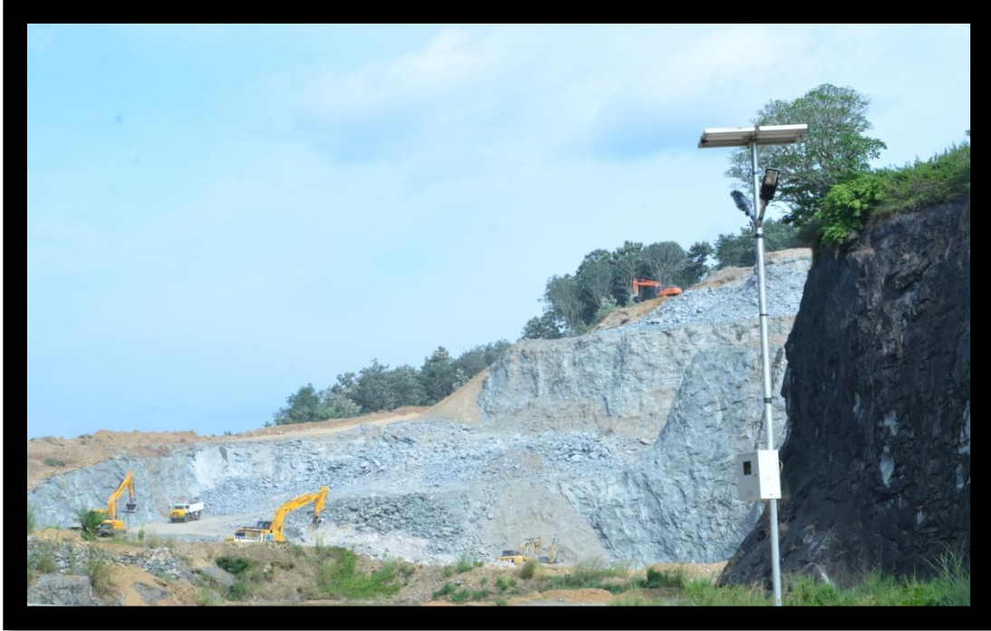
Solar Street light
