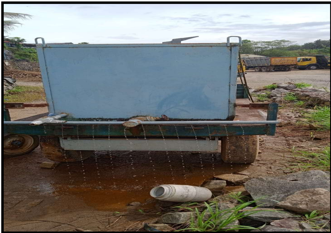
Wetting road using vehicle
