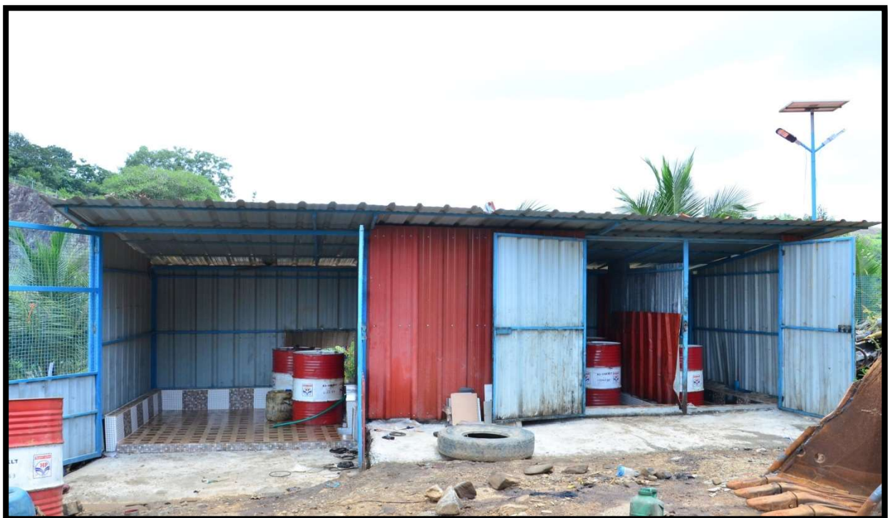
Used oil storage area
