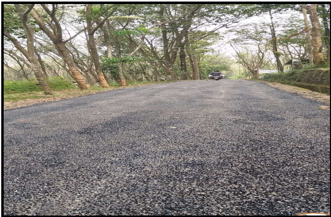
Tarred road to the quarry
