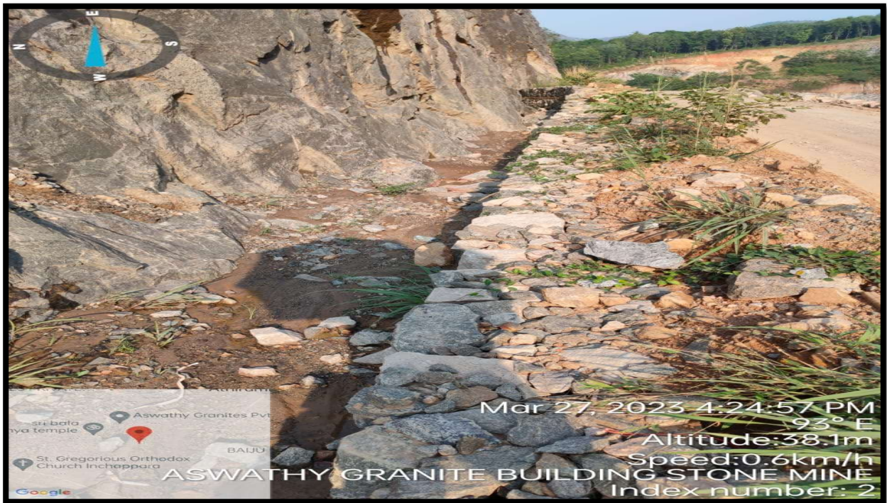
Periodic cleaning of silt traps
