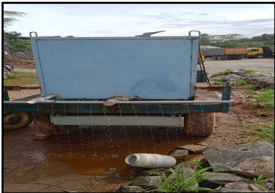
Wetting road using vehicle
