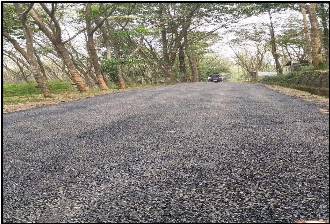
Tarred road to the quarry
