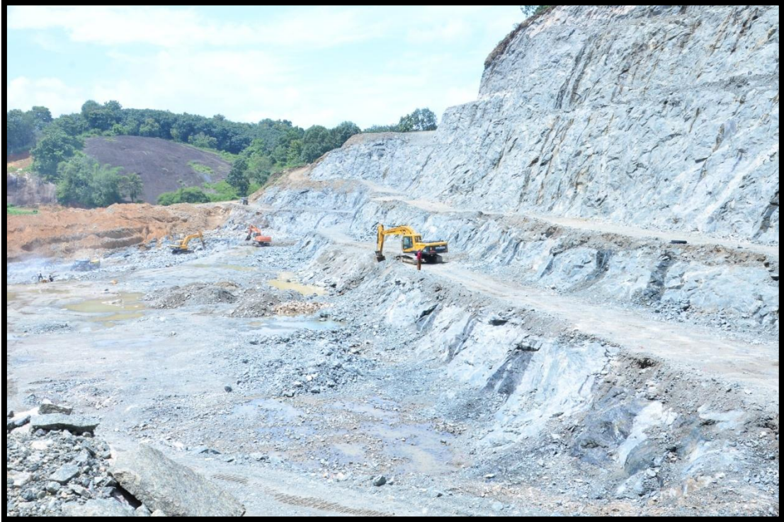
Benches under progress
