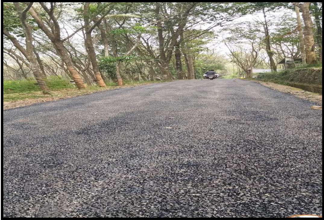
Tarred road to the quarry
