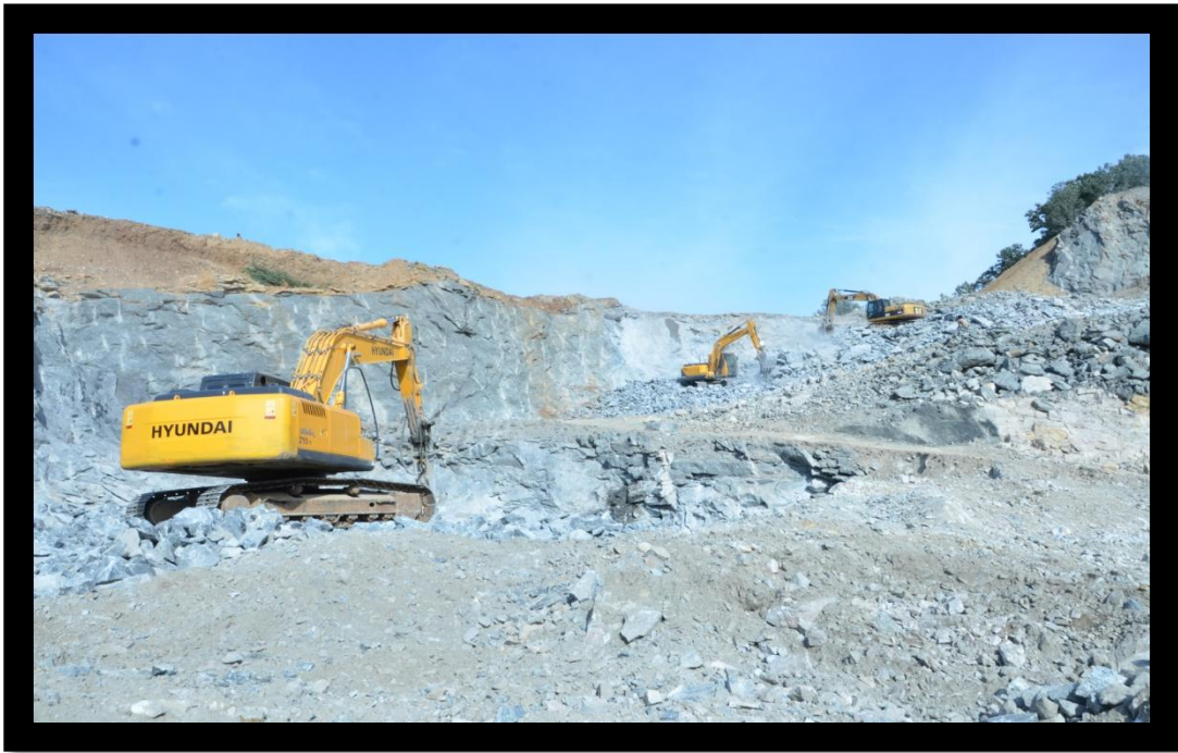
Benches under progress
