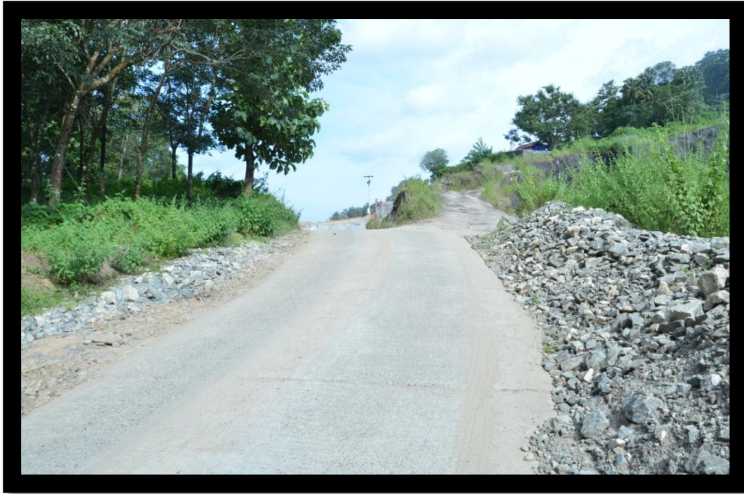
Concreted road to the quarry
